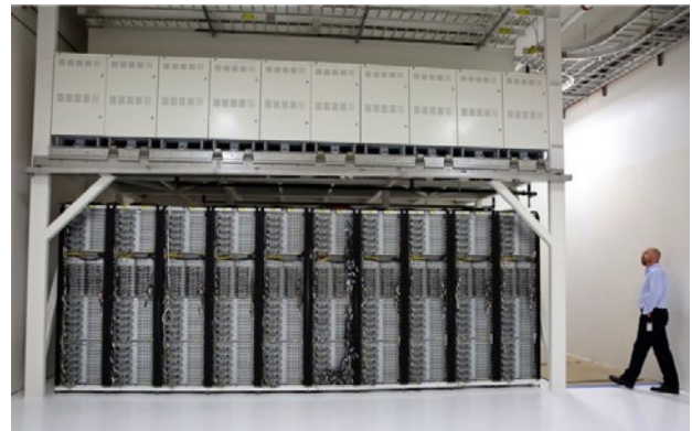
Figure 5 - Microsoft fuel cell on rack experimental data center 6
