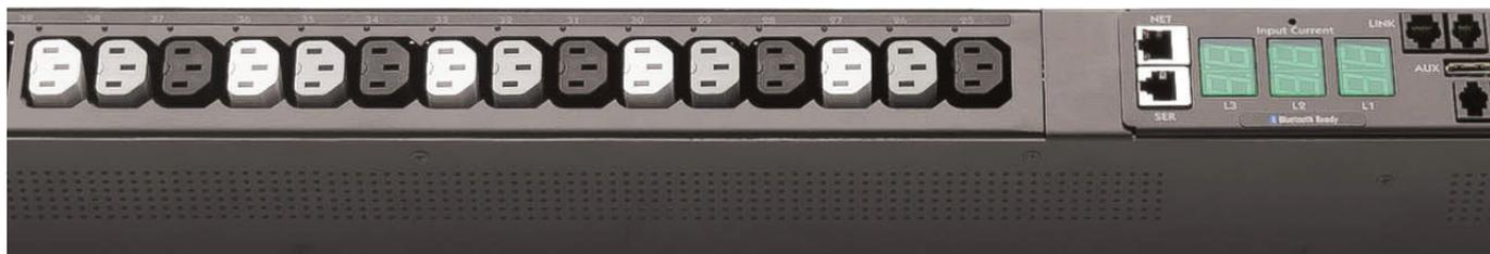
Outlets are grouped together up and down the PDU instead of broken up into individual branches.
