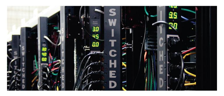
reboot stuck servers without the need for a trip to the colocation facility or calling for "remote hands" to manually go and cycle power on the server. "It only takes one or two instances of a locked up server being remotely reset to pay for the functionality of a Switched PDU," says Michael.
